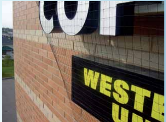
Bird netting was installed over signage to block birds from landing.
