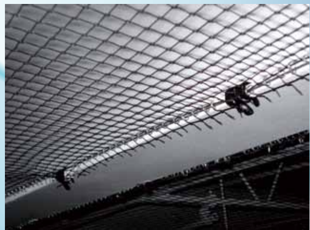
Girder Clips were used to secure the netting along the perimeter.
