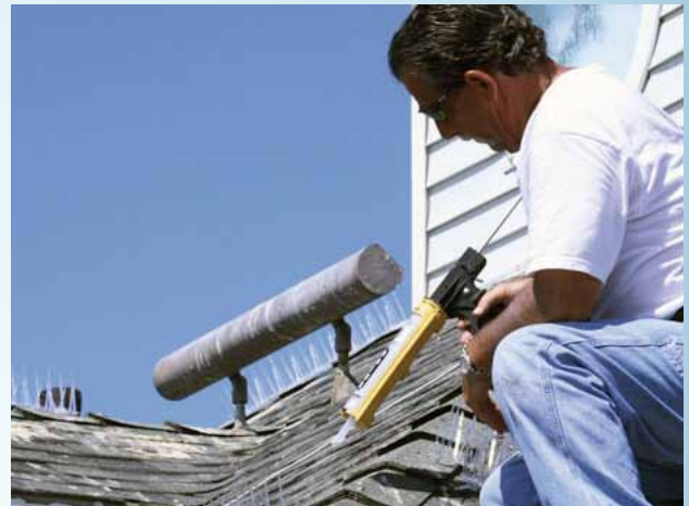
Bird Spikes can be easily installed with adhesive, screws or tie downs.
