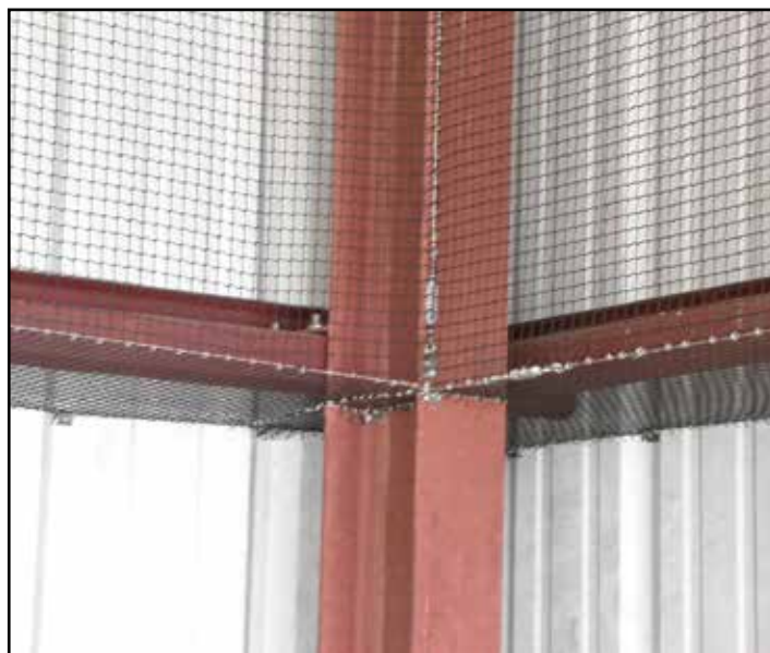
No-Knot Net on an interior I-beam
