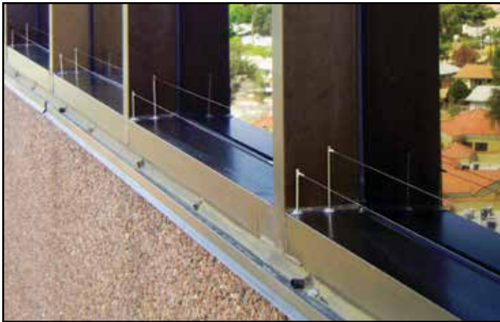
Bird Wire installed on window ledges
