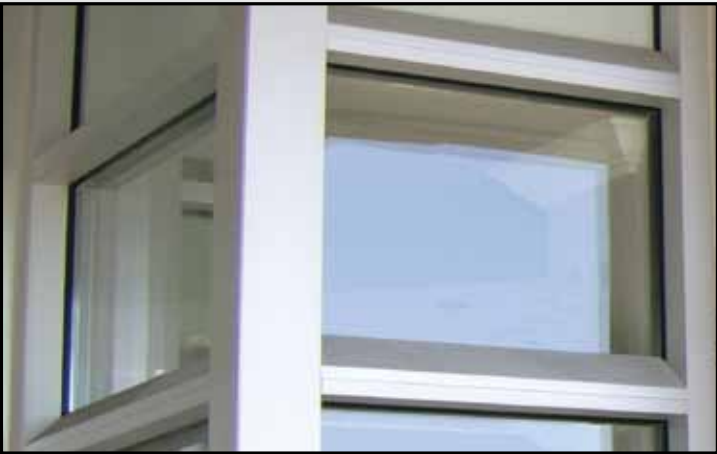
Bird Slope installed on window sills
