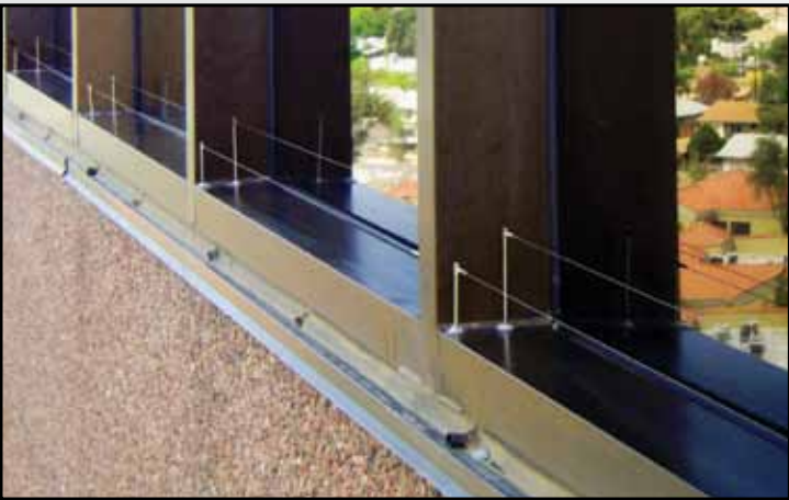
Bird Wire installed on window ledges
