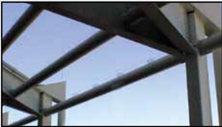
Custom Bird Wire brackets manufactured at Bird•B•Gone, installed on beams at the Orange County Convention Center, Orlando, FL.
