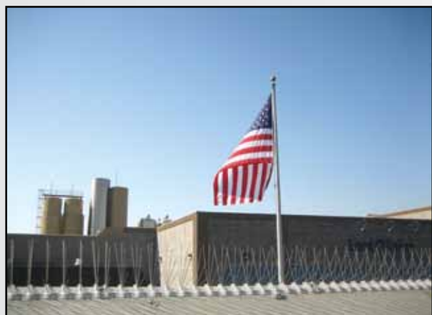
Stainless Steel bird spikes installed on a parapet.
