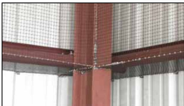
No-Knot Net on an interior I-beam
