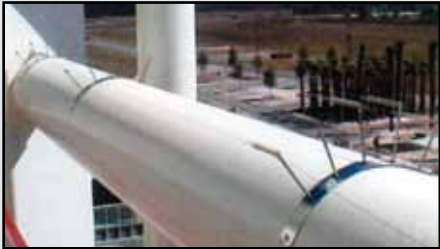
Custom Bird Wire brackets manufactured at Bird•B•Gone, installed on beams at the Orange County Convention Center, Orlando, FL.
