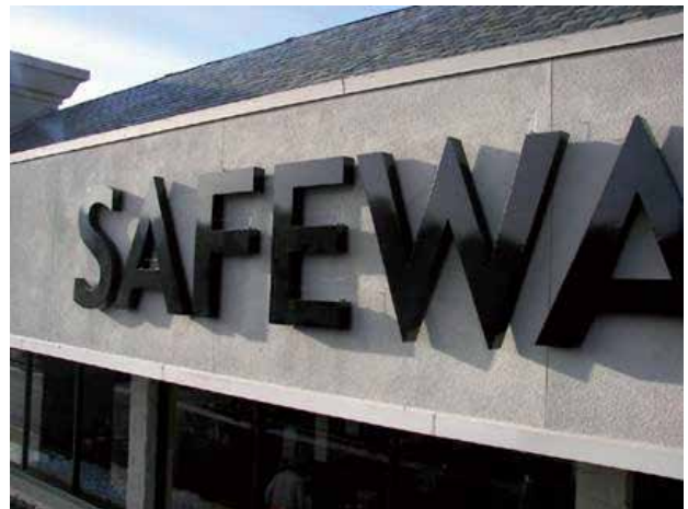
With all of the bird deterrents had been installed, they were virtually invisible.
