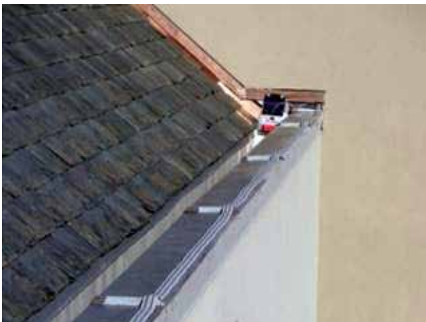
Bird Jolt Flat Track™ was installed to keep birds off the parapet walls and ledges.
