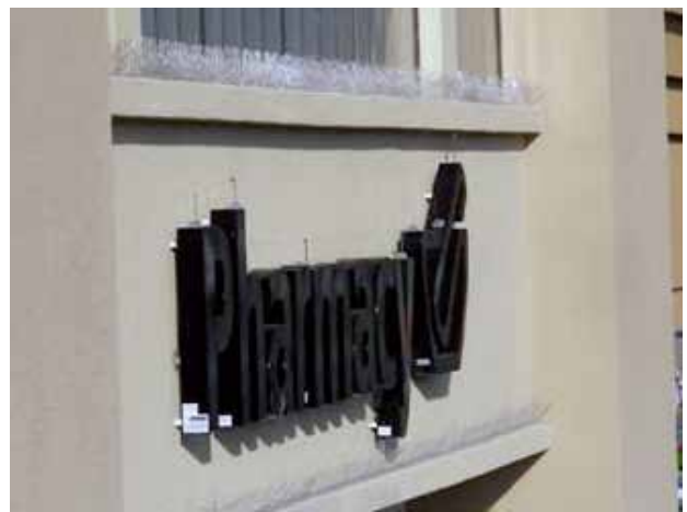
Bird Spikes were installed on the window ledge directly above the sign.
