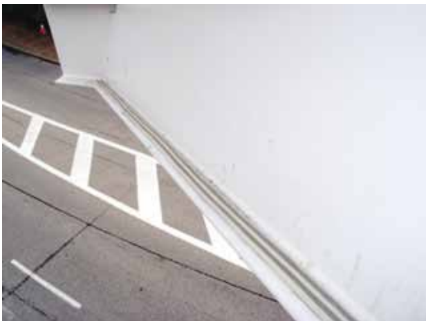
Bird Jolt Flat Track™ was installed using adhesive to glue it down to the ledges and beams.
