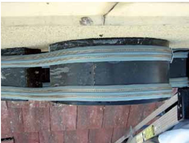
Bird Jolt Flat Track® is flexible and conforms to the shape of each channel letter.
