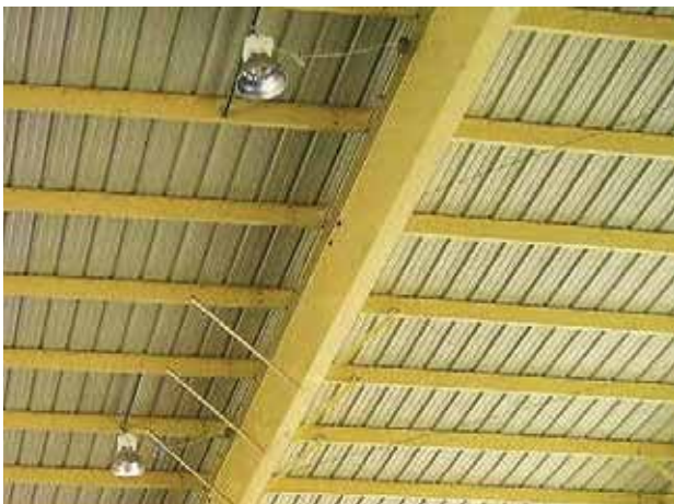
The bird netting was installed onto existing beams with girder clamps and straining wire.
