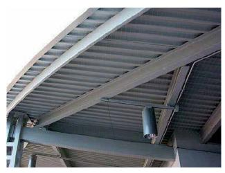
Bird Netting was installed under the beams as a barrier to block birds.
