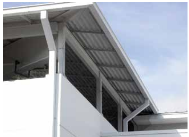
Netting was installed vertically along the backside to prevent birds from entering.
