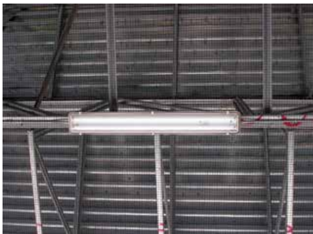
Bird Netting was wrapped around light fixtures to allow access.
