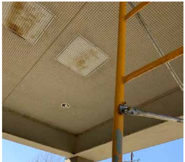
Virtually invisible once installed, bird netting keeps swallows from returning to the area.
