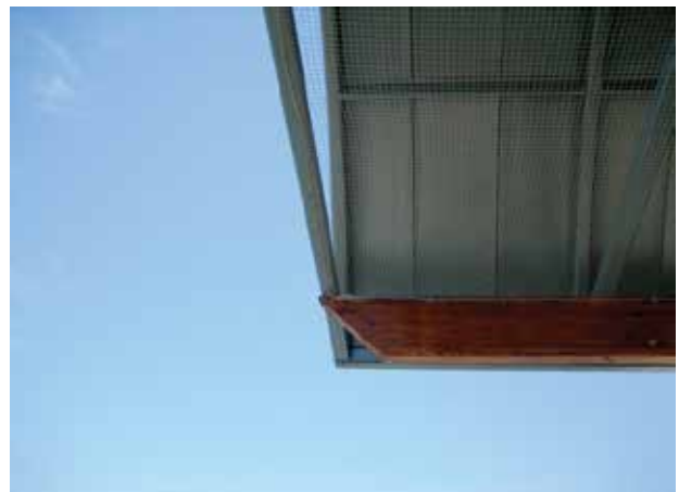
The stone colored bird netting blended well with the canopy for a low profile solution.
