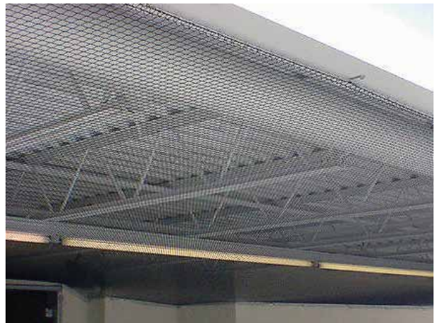
Bird Netting was also installed to prevent birds from nesting above the loading dock.
