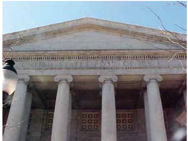
The high profile historic building required a low profile bird deterrent.
