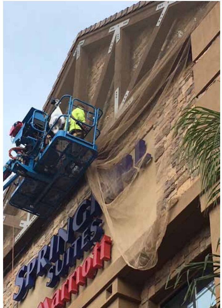
Installation of Bird•B•Gone® Heavy Duty Bird Netting.
