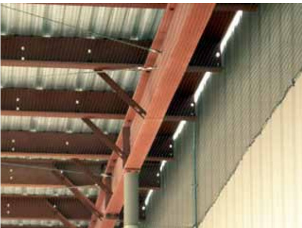
Bird Net 2000™ was installed to block birds from sitting on I-beams.
