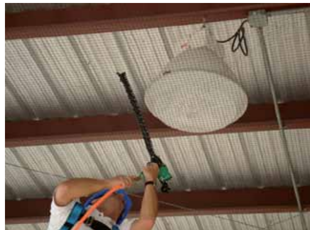
Zipper can be installed in bird netting to allow access to features such as light fixtures.
