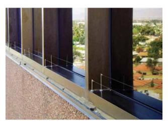
The Bird Wire system is a low cost, maintenance free bird deterrent system.
