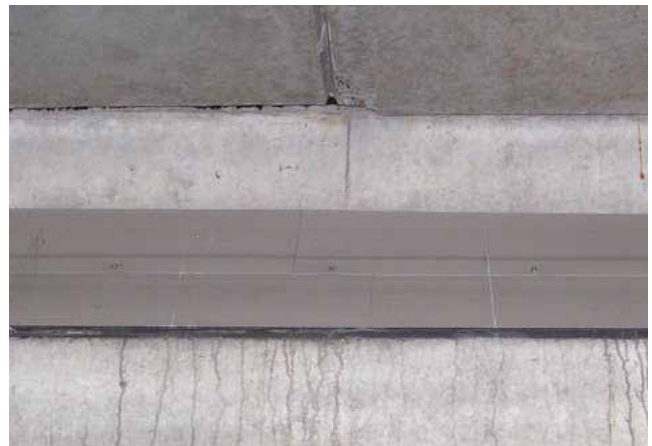
Bird Slope™ Extenders were installed to cover wide ledges and will extend slope up to 10".
