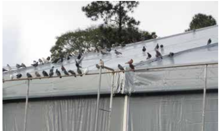
Before installation of Bird•B•Gone® Polycarbonate bird spikes.
