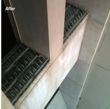
formulated adhesives were used to secure the spikes to the ledges. Result: no more pigeons or pigeon droppings on the ledges of this building.
