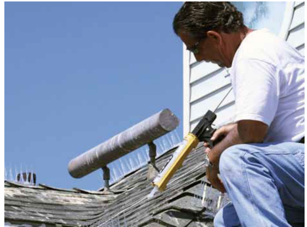
Bird Spikes can be easily installed with screws, tie downs, or adhesive.
