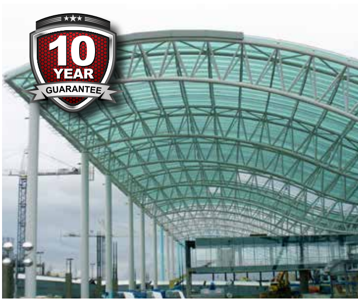
50,000 sq. ft. of Bird Net 2000™ installed at Gerald Ford International Airport
