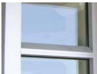
Installed on window sills
