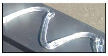
To install: Bird-OFF™ Gel is applied in a zig-zag pattern with no more than 2" (5 cm) gaps. Do not install on a vertical surface.
