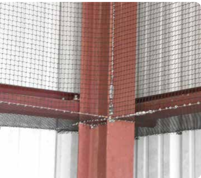
No-Knot Net on an interior I-beam
